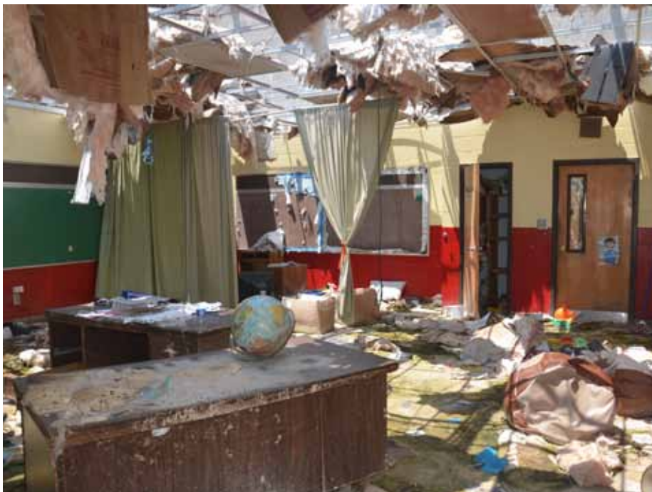
Hackleburg's elementary school was destroyed by the EF-5 tornado on April 27 th . (Photo by Carrie Banks)
